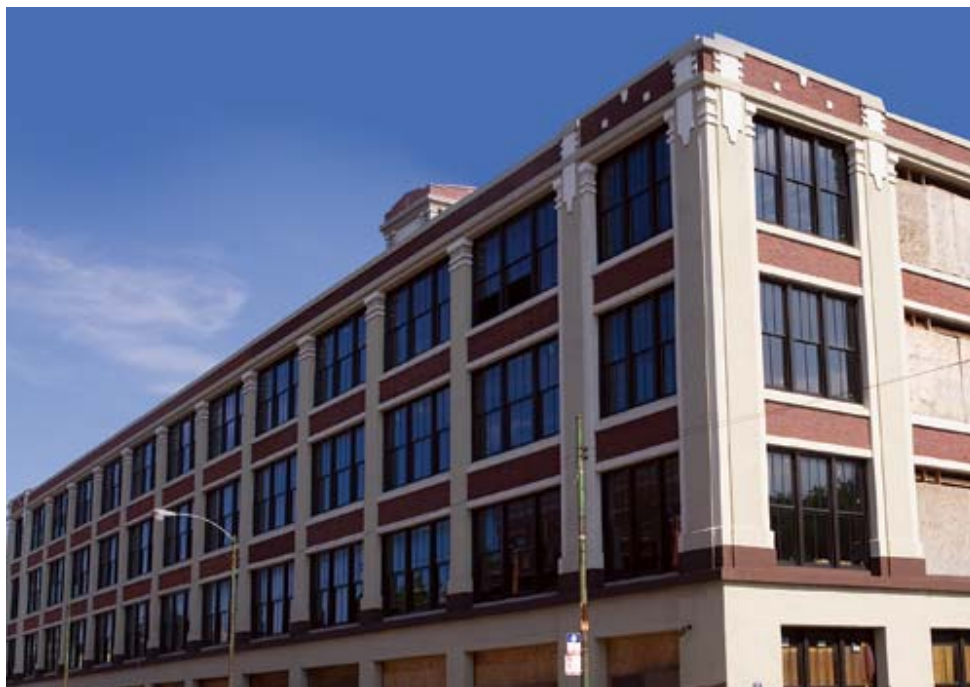
The Green Exchange at 2545 W. Diversey Ave.
